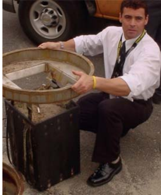
Westchester County Airport's Parletta removes an AbTech Ultra-Urban Filter for inspection.
